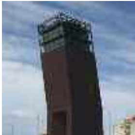
Port of Barcelona control tower / Shipping traffic control system / Autonomous Port of Barcelona.
